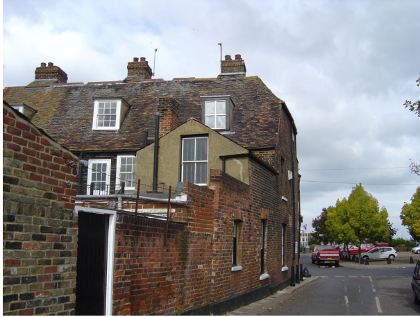
Plate 2 Rear elevation of 9 High Street Queenborough showing second floor PVCu window to be replaced with timber sash.
