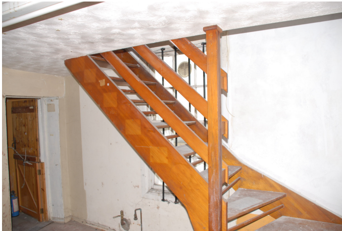
Plate 3 Upper part of existing internal stair to be removed.
