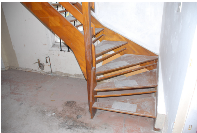
Plate 4 Lower part of existing internal stair to be removed.
