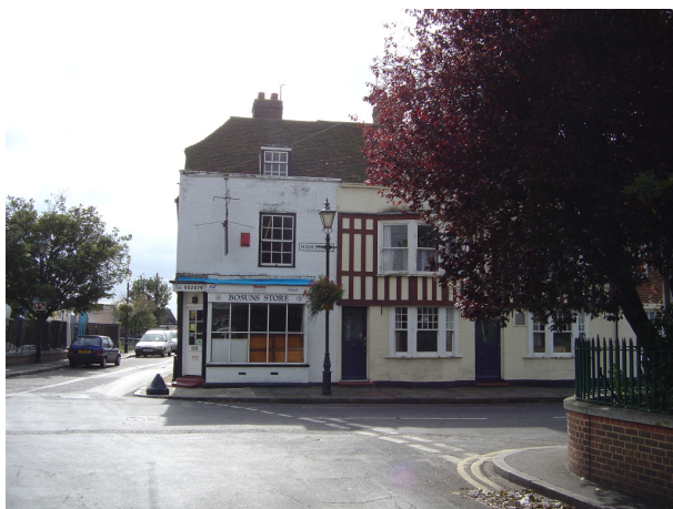
Plate 1 Front elevation of 9 High Street Queenborough.
